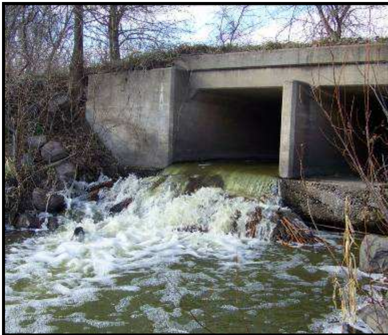
Outlet Structure of High Island Lake (11/17/2008)
