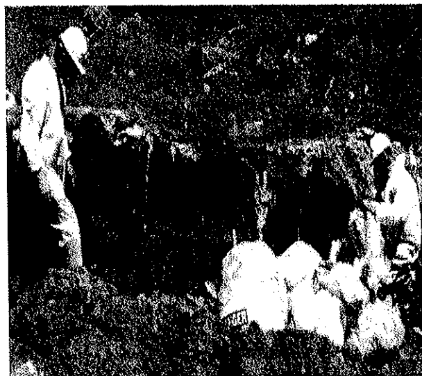
Licensed contractors removing asbestos waste material from a site near the University of Minnesota in Minneapolis
